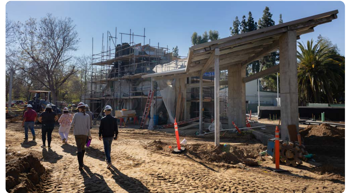
Photos show the construction progress for Zooplex and Kingdoms of Asia
